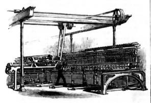
considered that these spindles and flyers revolve from 1000 to 2000 times in a minute, the perfection with which they must be finished and hardened, in order that they may move steadily and without self-destruction, and the consumption of power, may be easily conceived.
