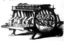
Our drawing represents the winding machine as made Mr. Frost of Macclesfield, the skeins of raw silk are put on the swifts which are six-armed reels, with string cross h to form the fork in which the skein lies. The axles of swifts lie loosely in centres, and the framing descends lower than this centre, so that there is very little liability knocking. The thread is passed through glass guit arranged on a traversing guide bar, to the bobbins.
