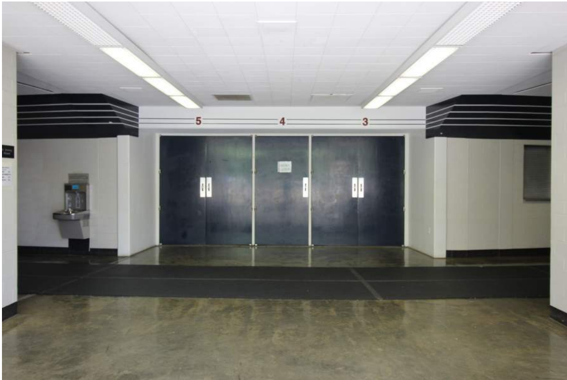
DHR Identification Number: 104-5292 June 4, 2018 Quinn Evans Architects 253 northeast entrance, looking southwest.
