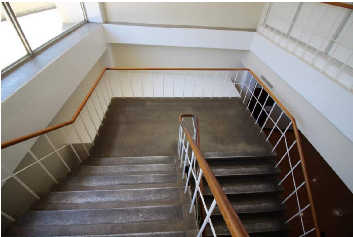
DHR Identification Number: 104-5292 June 4, 2018 Quinn Evans Architects 250 east stair, public level, looking east.
