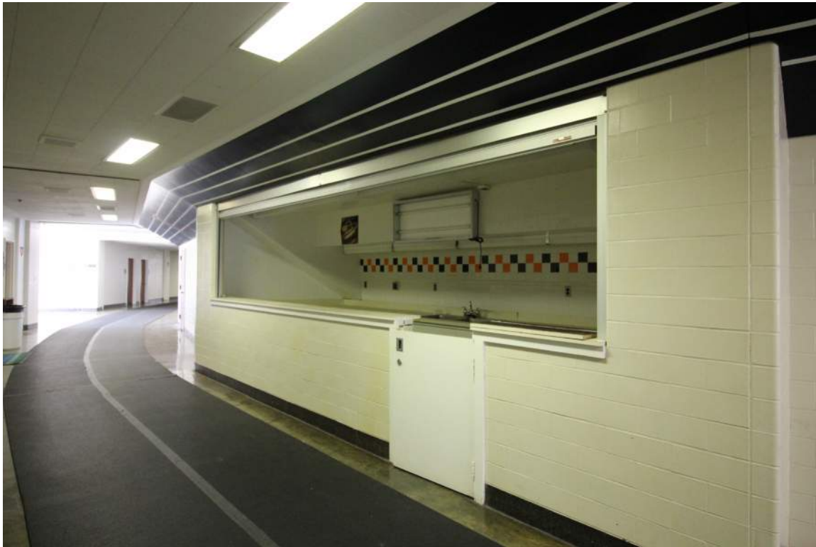
DHR Identification Number: 104-5292 June 4, 2018 Quinn Evans Architects 259 concession stand, looking southwest.
