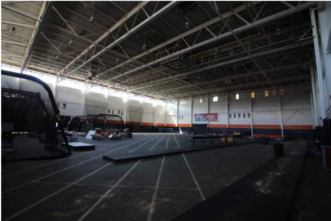
DHR Identification Number: 104-5292 June 4, 2018 Quinn Evans Architects Cage interior looking southeast.
