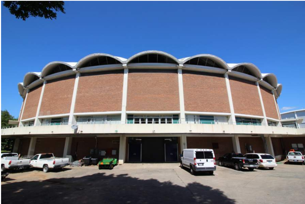
DHR Identification Number: 104-5292 June 4, 2018 Quinn Evans Architects Southwest elevation and service parking lot, looking northeast.
