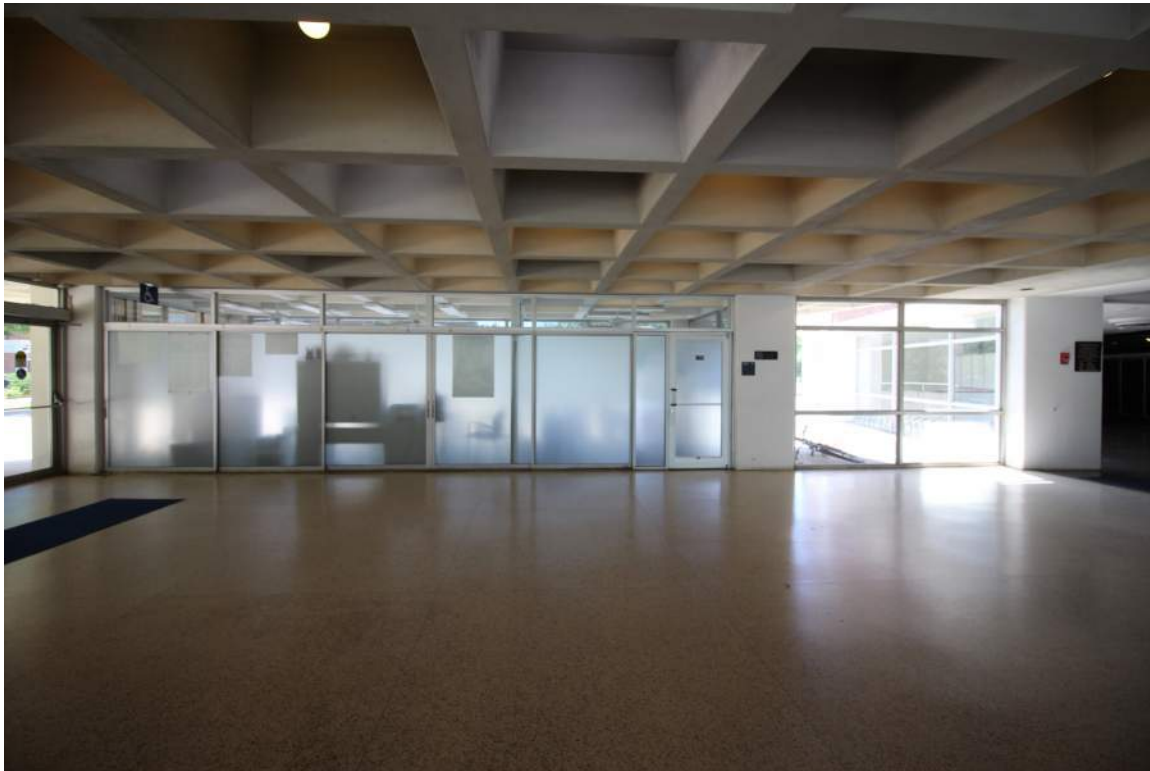
DHR Identification Number: 104-5292 June 4, 2018 Quinn Evans Architects 248 main entrance lobby, looking east.
