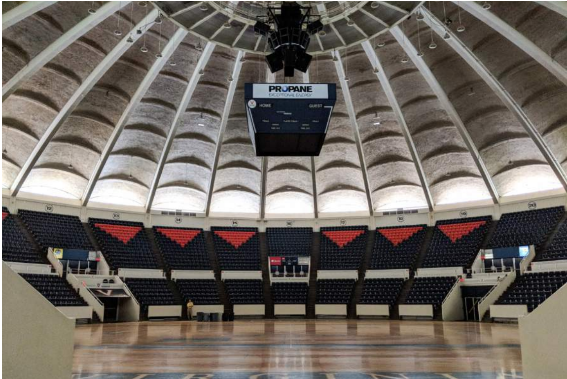
DHR Identification Number: 104-5292 June 4, 2018 Quinn Evans Architects Arena, view from north player level entrance.
