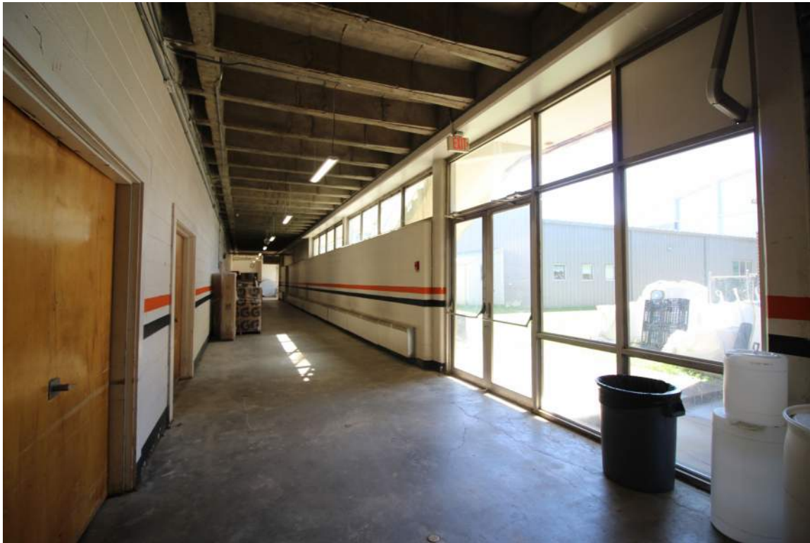
DHR Identification Number: 104-5292 June 4, 2018 Quinn Evans Architects 153 link corridor, looking northeast.
