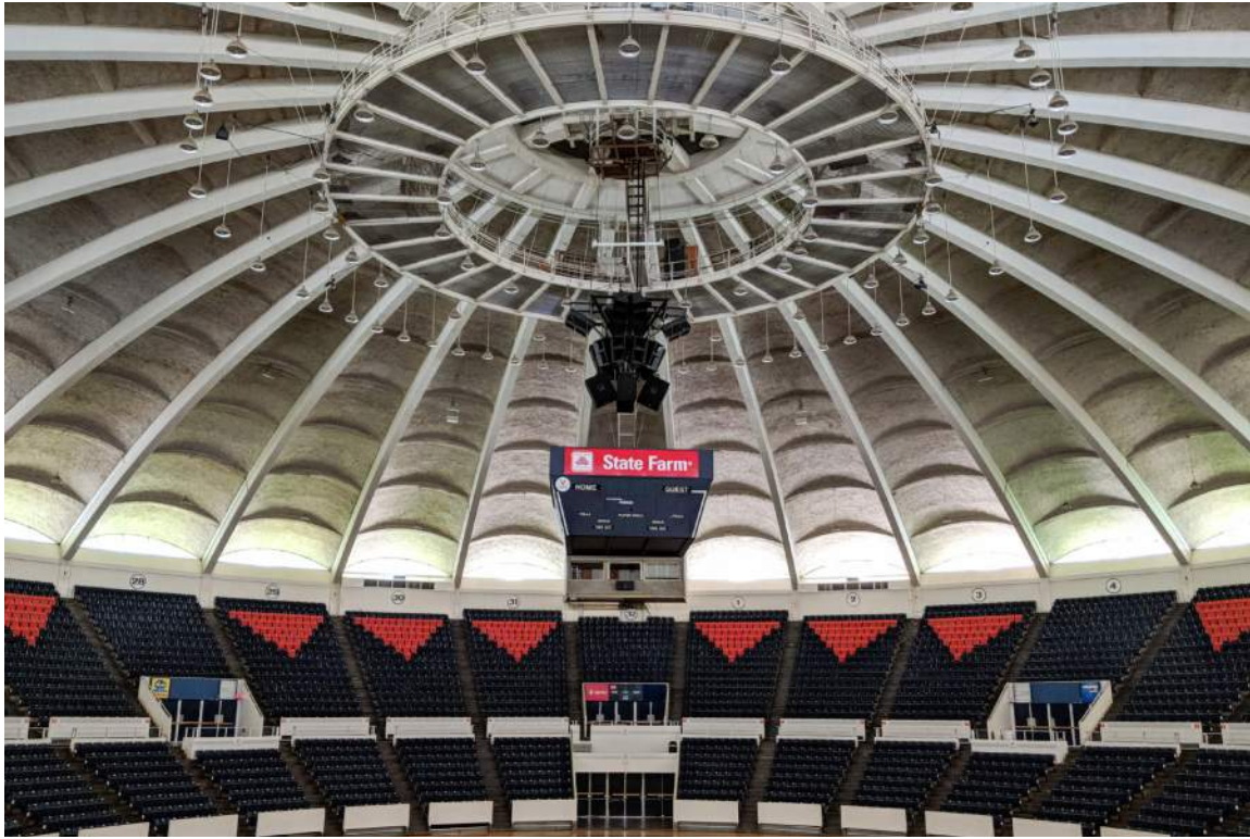
DHR Identification Number: 104-5292 June 4, 2018 Quinn Evans Architects Arena, looking north from the center aisle.
