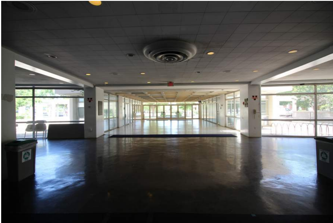
DHR Identification Number: 104-5292 June 4, 2018 Quinn Evans Architects 250 north entrance lobby, looking north.
