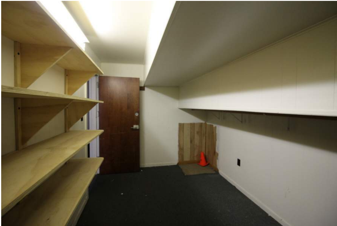
DHR Identification Number: 104-5292 June 4, 2018 Quinn Evans Architects 205 storage, looking southeast.
