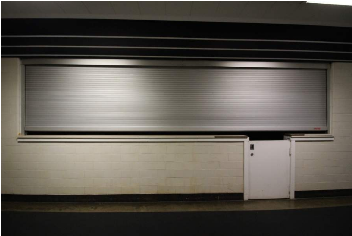
DHR Identification Number: 104-5292 June 4, 2018 Quinn Evans Architects 239 concessions stand, looking east.
