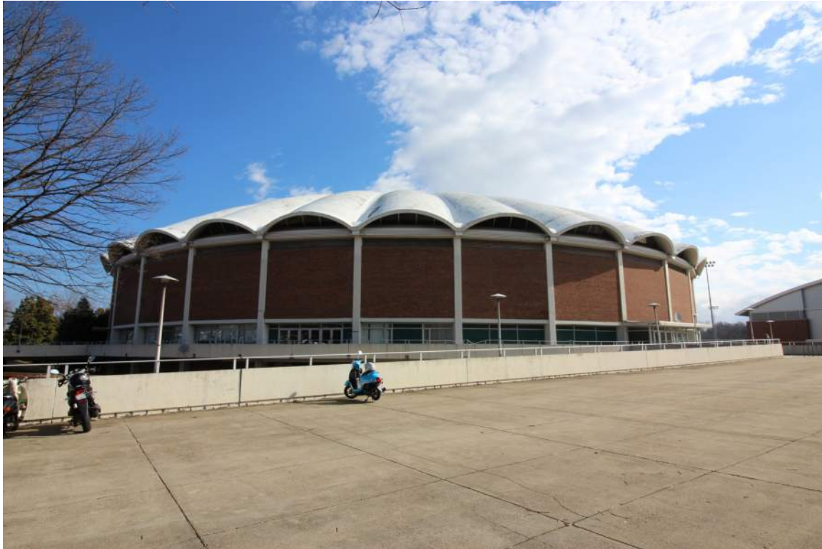
DHR Identification Number: 104-5292 June 4, 2018 Quinn Evans Architects Ramp to south entrance plaza, looking northeast.
