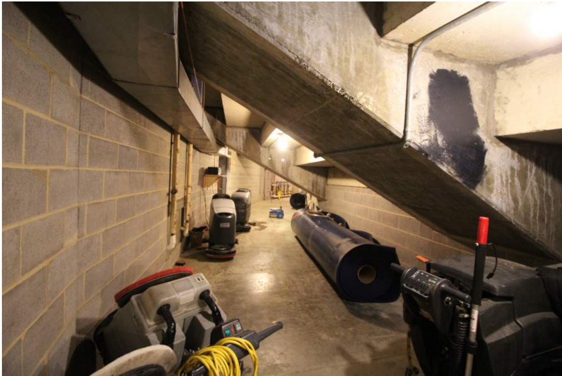
DHR Identification Number: 104-5292 June 4, 2018 Quinn Evans Architects 114 Storage, looking west.
